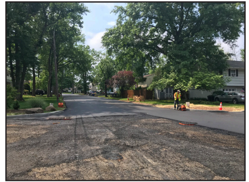
FIGURE 1.6. Madison Avenue Road Repairs
