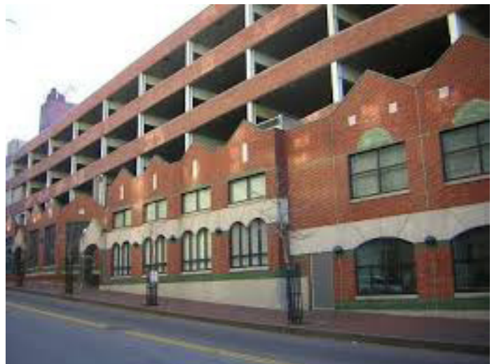
FIGURE 5.2. Structured parking erected above historic building in Portland, OR.
