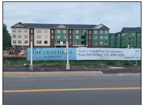
FIGURE 2.1. Dunellen Station Project, Under Construction
