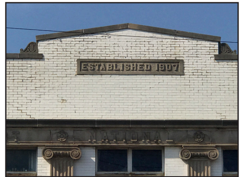
FIGURE 1.7. Historic architectural features
