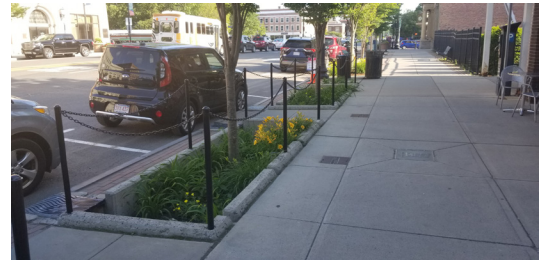
FIGURE 4.12. Sidewalk bioswales in Pittsfield, MA
